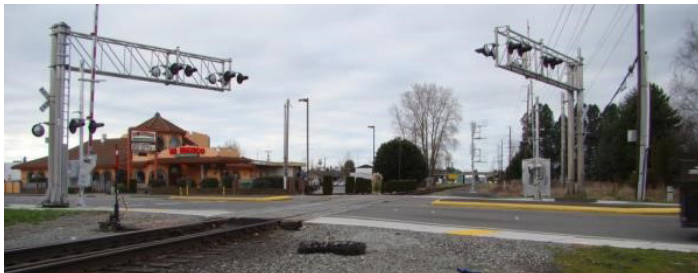
Example of an at-grade crossing (intersection of South Burlington Boulevard/Anacortes Subdivision, looking southwest)
