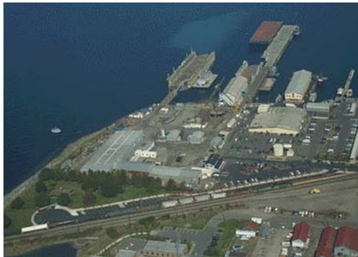
The Harris Avenue Shipyard site is on the southern shore of Bellingham Bay in Fairhaven.
