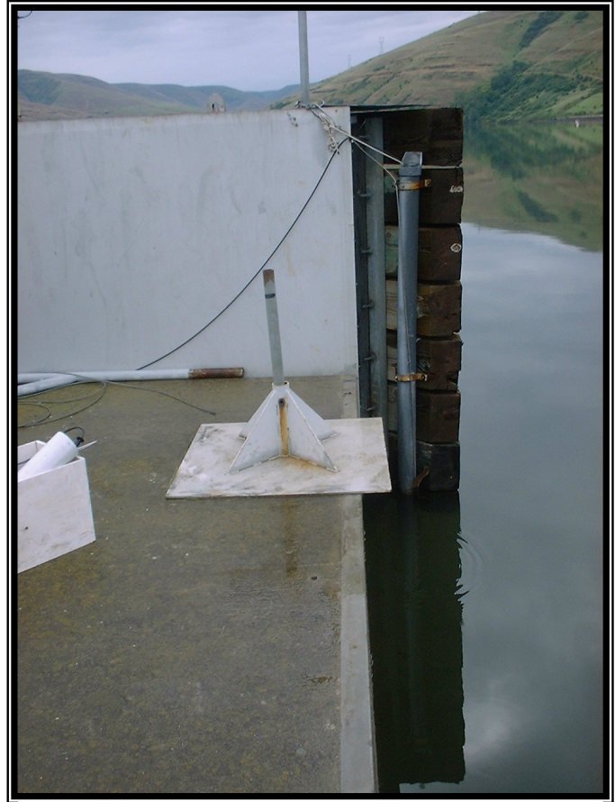
Figure 2. TDG continuous monitoring deployment with a PVC pipe mounted from a bulkhead.
