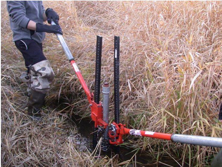
Figure 12 - Decommissioning a steel piezometer with high-lift jacks
