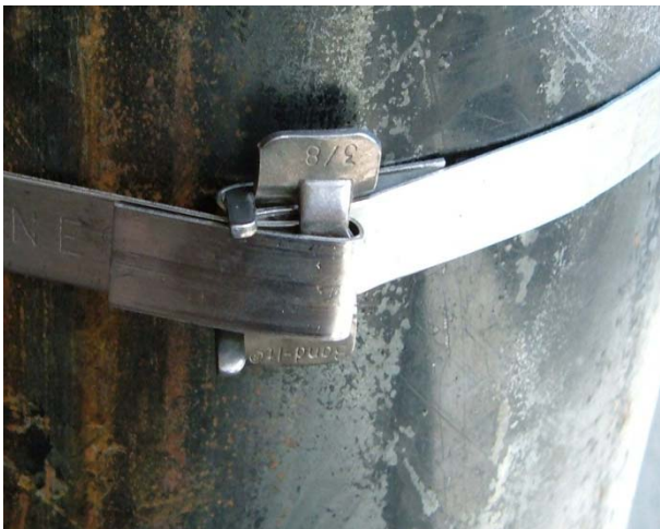
Figure 10 A. Locking the band
