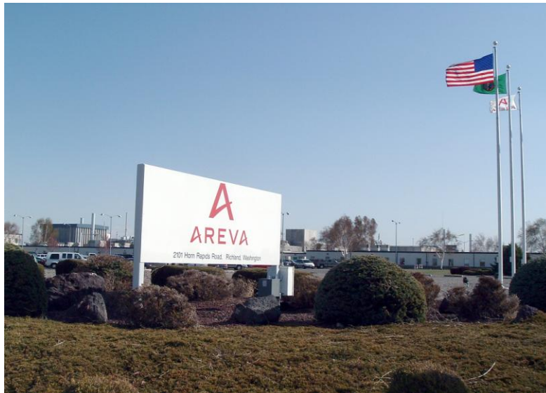
AREVA's Nuclear Fuel Fabrication Plant at 2101 Horn Rapids Road, Richland WA 99354
