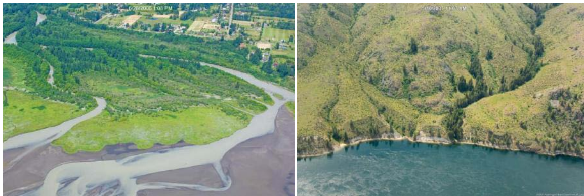
Figure 13-9: The Natural environment designation is applied to the mouth of the Nooksack River in Whatcom County (left) and on the Douglas County side of the Columbia River west of Nespelem Bar. (Washington Coastal Atlas photos.)
