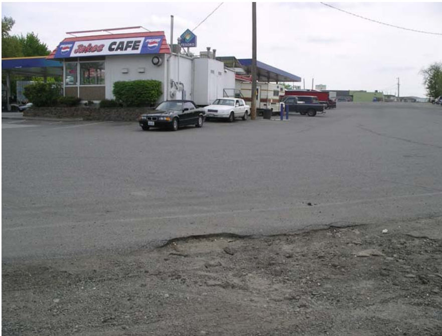
Photo 2: Back of store – from the northwest
