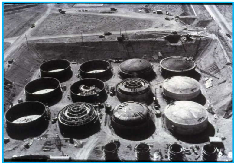
C-Farm tank construction, 1944.
